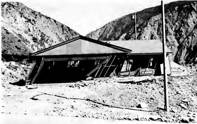
Photo 9. Partially completed structure with a good portion of sheathing and wire mesh placed. Rajah Street and Tucker Avenue area. Photo courtesy of the City of Los Angeles Department of Building and Safety.
